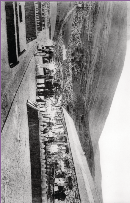
The Lower Mill, looking east with the Beudynewydd Incline in the left background and the slate stacking area prominent in the foreground. The bridge carrying the tramway for the waste stone across the Incline is visible. The waste tips would eventually grow to be very much larger. The roof just visible above the workmen is that of Beudybach (The Little Cowshead), a building that would eventually be swamped by the growing waste tip. It was replaced by Beudynewydd (New Cowshead) Farm. Credit TR Collection.
